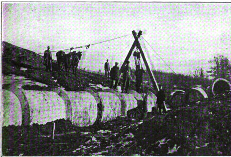
Laying a 48-In. Concrete-Pipe Culvert
